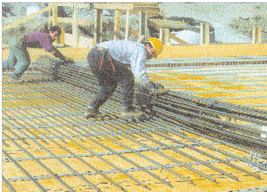
Two workers are enough to unroll the mat onto the formwork.
