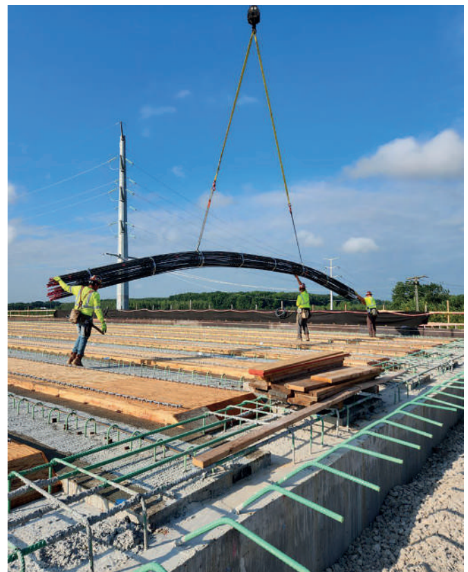
First BAMTEC ® Bridge Deck, Ohio, USA
