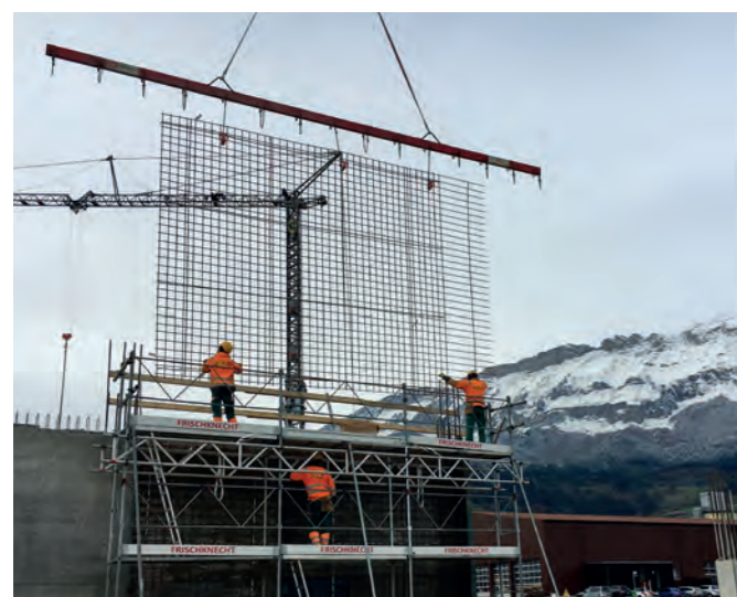
BAMTEC® WALL application in Switzerland
