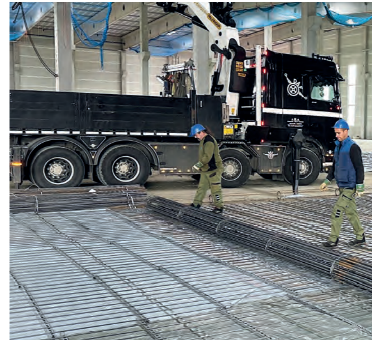
BAMTEC® Installation
